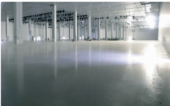
Figures 1 and 2: The size of the Distribution Centre in Corby lent itself to jointless panel sizes 30 × 30m with no sawn contraction joints at all.
